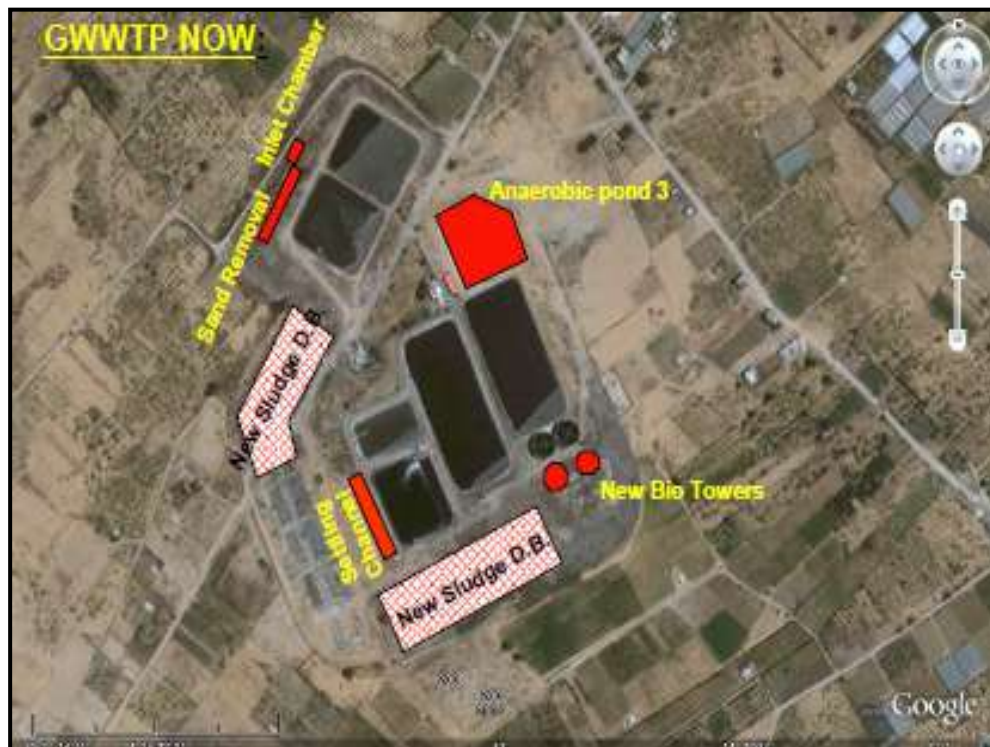
Figure 3.3: Aerial Photo of the Gaza City Wastewater Treatment Plant (CMWU, 2012).
