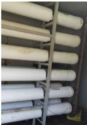
Figure 17: Photos of BWRO desalination unit in Maraj Na'aja
