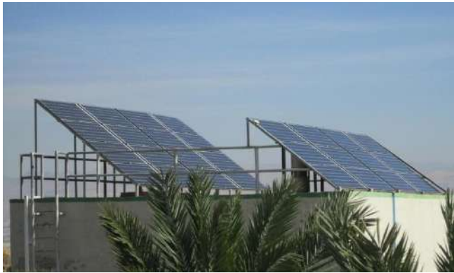
Figure 19: Photo of the PV arrays in Al- Zubiedat BWRO dealinatio unit, (Yousef, 2013)
